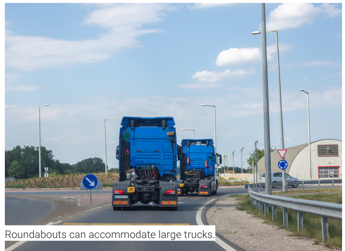
Example of a roundabout.
