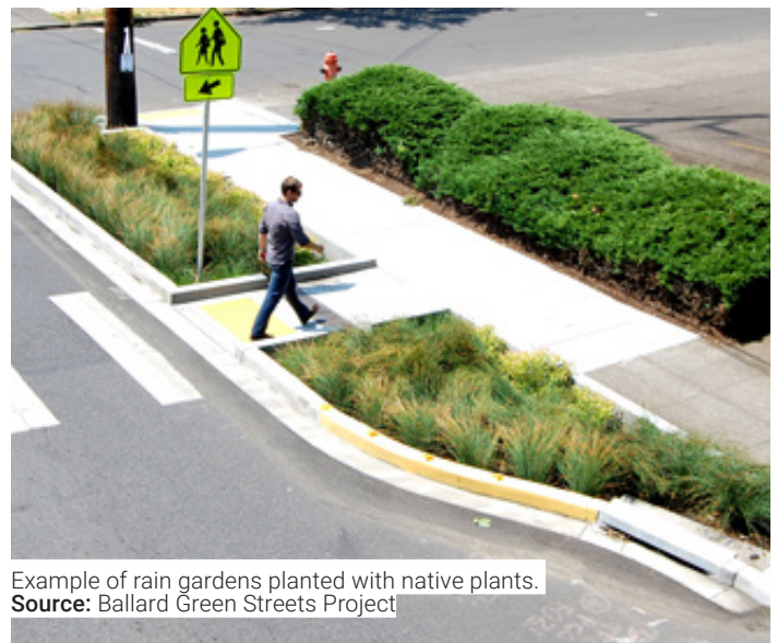
Example of a bioswale integrated into a suburban street.
