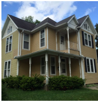
FIGURE 6: 117 EAST OAK STREET. THIS THREE-QUARTERED VIEW FROM THE STREET SHOWS PROTRUDING BAYS, A WRAPAROUND PORCH AND SPINDLE WORK COLUMNS, IRREGULAR WINDOW STYLE, AND WHITE DORMER TRIM.
