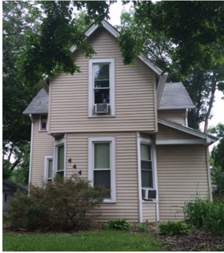
FIGURE 14: ANOTHER VERNACULAR FORM IS THE T-PLAN, WHEREIN THE AERIAL PLAN WOULD SHOW A CROSSED "T" SHAPE. 444 NORTH SALISBURY STREET (C. 1890)
