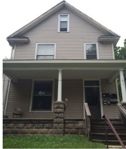
FIGURE 15: THE SYMMETRICAL SIMPLICITY OF THE GABLE-FRONT HOME AT 411 NORTH SALISBURY STREET (C. 1915)
