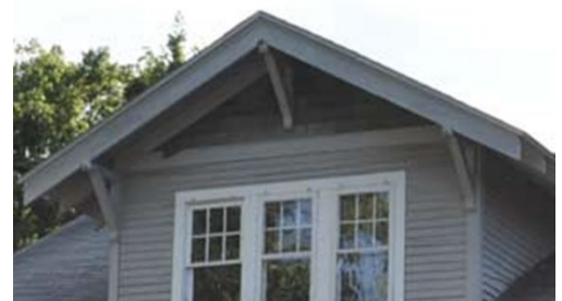
FIGURE 22: AS SEEN HERE, WINDOWS ARE INTEGRAL TO THE HISTORIC STYLISTIC CHARACTER OF HOMES. THE CHARLES AND GERTRUDE RAWLS HOUSE, AT 545 HAYES STREET, HAS WINDOWS THAT UTILIZE MUNTIN DESIGN TYPICAL OF CRAFTSMAN BUNGALOW—THREE DIVIDED LIGHTS OVER ONE.
