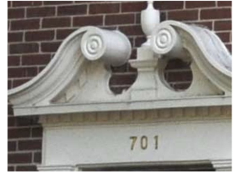
FIGURE 21: FAÇADE DETAILS, AS SHOWN HERE AT THE JOHN AND JEAN BRAY HOUSE AT 701 N. CHAUNCEY, CONTRIBUTE TO ITS OVERALL HISTORIC CHARACTER AND STYLE (COLONIAL REVIVAL). THE SCROLLS HERE ARE TYPICAL OF CLASSICAL DETAILS SEEN IN COLONIAL REVIVAL ARCHITECTURE.
