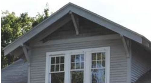
FIGURE 22: AS SEEN HERE, WINDOWS ARE INTEGRAL TO THE HISTORIC STYLISTIC CHARACTER OF HOMES. THE CHARLES AND GERTRUDE RAWLS HOUSE, AT 545 HAYES STREET, HAS WINDOWS THAT UTILIZE MUNTIN DESIGN TYPICAL OF CRAFTSMAN BUNGALOW—THREE DIVIDED LIGHTS OVER ONE.
