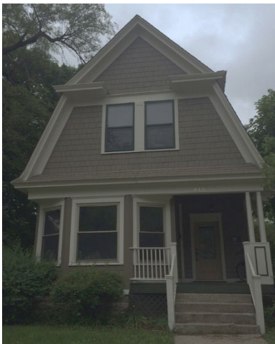
FIGURE 11 : A GAMBRELED ROOF MARKS THE COLONIAL REVIVAL HOME OF 439 NORTH SALISBURY ST. (c. 1915)
