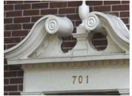
FIGURE 21: MASONRY DETAILS, AS SHOWN HERE AT THE JOHN AND JEAN BRAY HOUSE AT 701 N. CHAUNCEY, CONTRIBUTE TO ITS OVERALL HISTORIC CHARACTER AND STYLE (COLONIAL REVIVAL). THE SCROLLS HERE ARE TYPICAL OF CLASSICAL DETAILS SEEN IN COLONIAL REVIVAL ARCHITECTURE.
