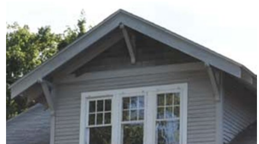
FIGURE 22: AS SEEN HERE, WINDOWS ARE INTEGRAL TO THE HISTORIC STYLISTIC CHARACTER OF HOMES. THE CHARLES AND GERTRUDE RAWLS HOUSE, AT 545 HAYES STREET, HAS WINDOWS THAT UTILIZE MUNTIN DESIGN TYPICAL OF CRAFTSMAN BUNGALOW—THREE DIVIDED LIGHTS OVER ONE.
