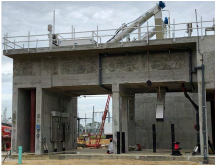
Construction of the new 4-mgd (expandable to 12-mgd) Northeast WRF began in 2022 using a construction manager at risk (CMAR) delivery method. Construction is on schedule to be completed in 2025.
